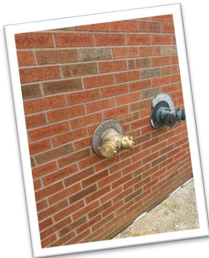
Replaced 42-year-old standpipe
